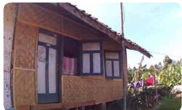
After the renovation.
