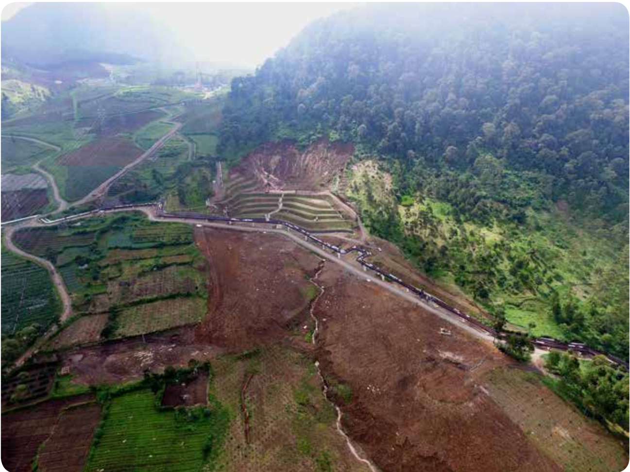
Conditions after reconnecting the pipeline, included constructing terracing, gabions, planting grass and trees where the landslide had occurred.
