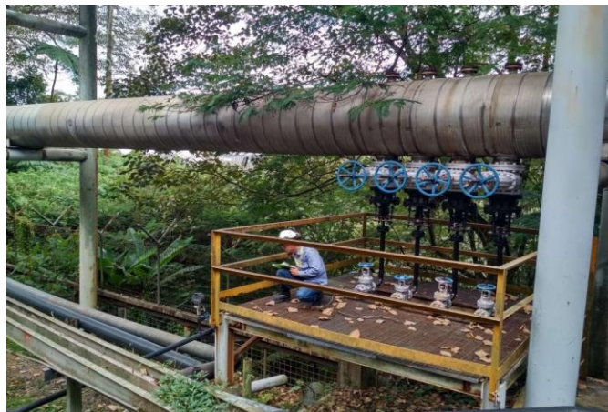
Gambar F4. Pengecekan Rutin Kegiatan Steam Wash Solid Particle Removal
